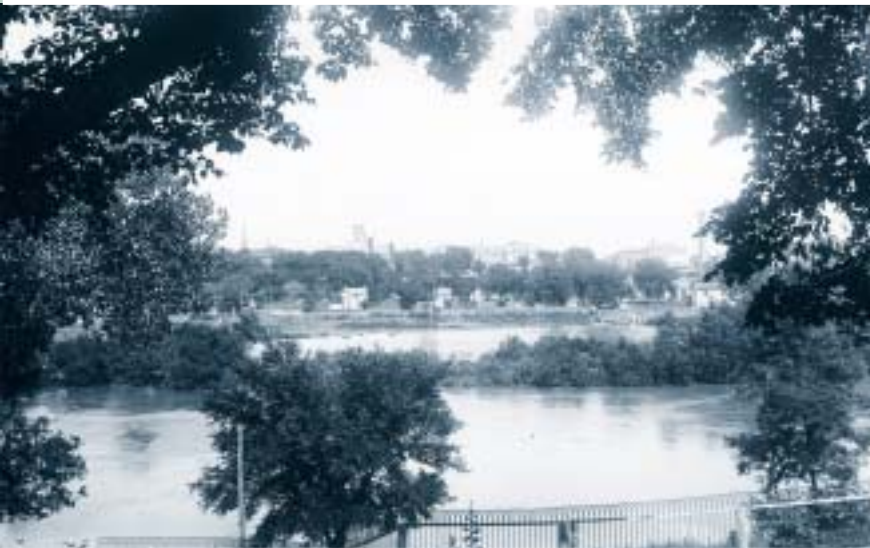
▼ WEST SIDE OF IOWA RIVER, HIGH WATER, IOWA CITY
