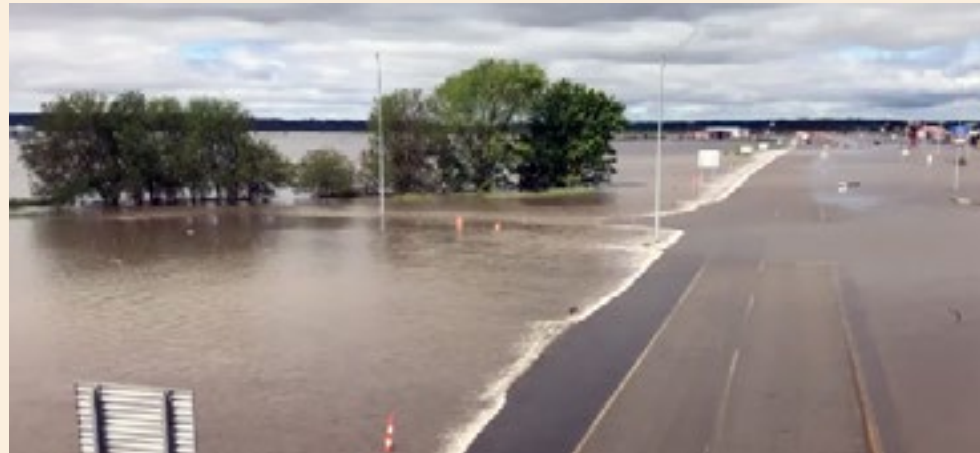
In early March a "bomb cyclone" and spring rains on frozen ground caused record flooding that closed Interstate-29.
