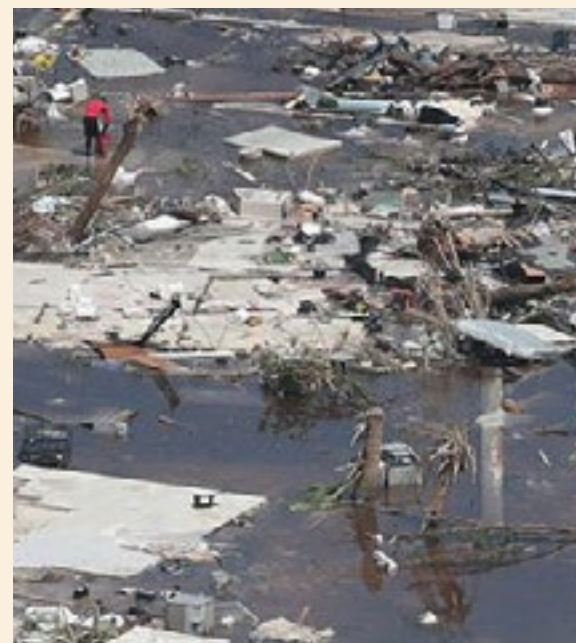
In September 2019, Hurricane Dorian caused extreme damage on Grand Bahama Island.
