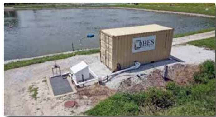
BES Water Solutions is working with IWWERP to optimize biological and physical-chemical treatment processes for small-town wastewater lagoons. The units can remove ammonia and suspended solids while providing pH adjustment and disinfection. Photo: Iowa Economic Development Authority.
