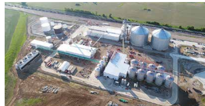
The wastewater treatment facility in Atlantic. Photo: Snyder & Associates.
