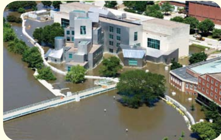
CGRER headquarters at the Iowa Advanced Technology Laboratories - one of twenty buildings on the UI campus to be affected by this summer's floods - were evacuated on June 13. Although first floor laboratories and office space suffered major damage, CGRER fortunately was saved by its location on fourth floor. The building will be reopened this autumn.
